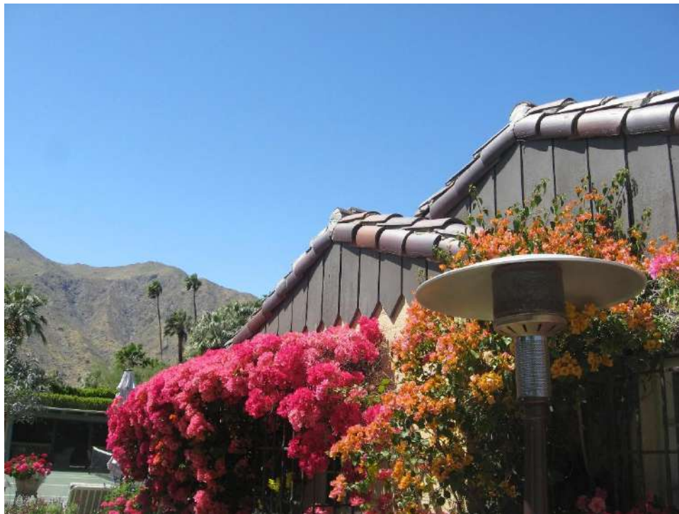
View west showing variegated roofs with sawtooth board cladding. (Author Photo. July 2023)
