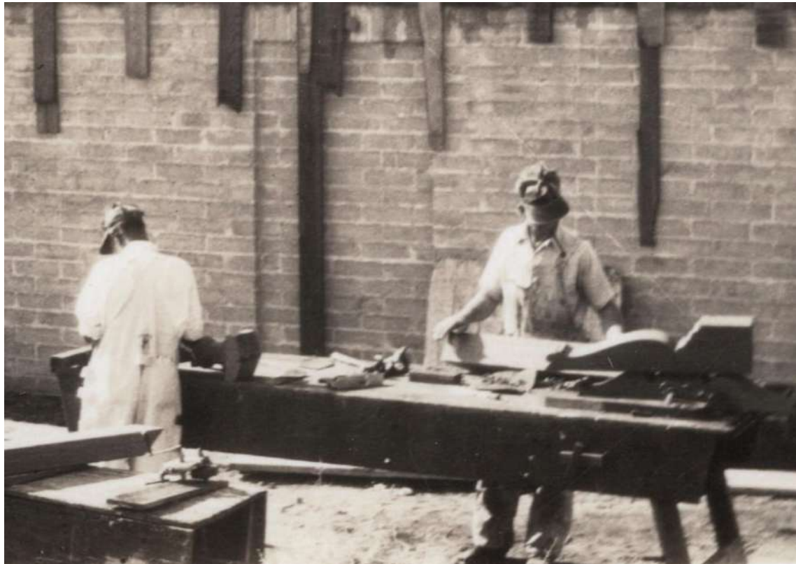
Skilled woodworkers preparing corbels for the living room beams on site ca. 1931. (Courtesy of Mary Kummings and Steve Scott)
