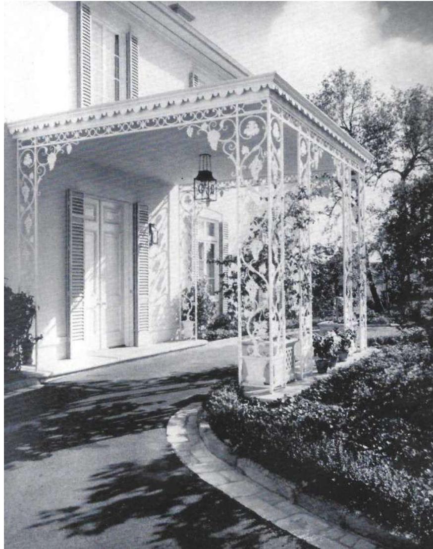
One of the unquestioned masters of Southern California Spanish architecture, Gordon B. Kaufmann, used wrought-iron in a similar fashion as Tanner, regularly including designs otherwise principally Spanish, Norman, Georgian, and English. This is an example from his 1938 Eugene Hill-Smith Residence in Holmby Hills, Los Angeles. (Via The Architectural Digest, Volume X, No. 3. 1940)
