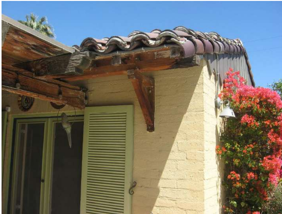
View facing east showing an eave brace and French doors to master bedroom. (Author Photo. July 2023)
