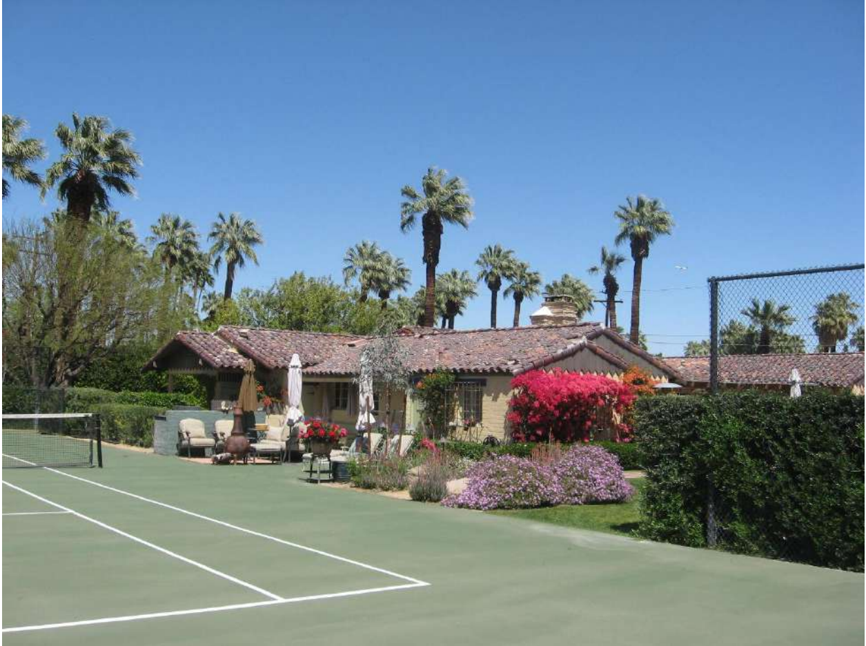
A recent (2023) image of the southern façade of Morada La Estrella (looking northeast) shows how Tanner varied roof heights to achieve a more interesting visual effect. Note, the sawtooth board cladding, a Tanner favorite, filling the gable ends. (Author photo. July 2023)
