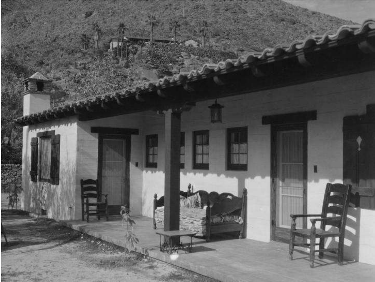
Part of a Desert Inn bungalow with Tanner's Ojo del Desierto presiding from above. Note the overall similarities with Morada La Estrella including the rustic chimney cap and the quartet of windows, a motif he also applied on Morada La Estrella's east façade. Lintels and the wooden porch columns/corbels are also shared attributes. (Courtesy Mott/Merge Collection. California State Library)
