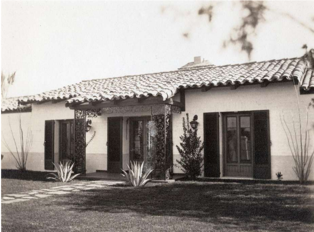
A 1930s view of a portion of Morada La Estrella's north (front) façade showing the main entrance flanked by what appear to be French doors on either side. These, however, were actually windows designed to match the look of the front door. Although not easy to see, there are brick lintels over the entry door and windows.
