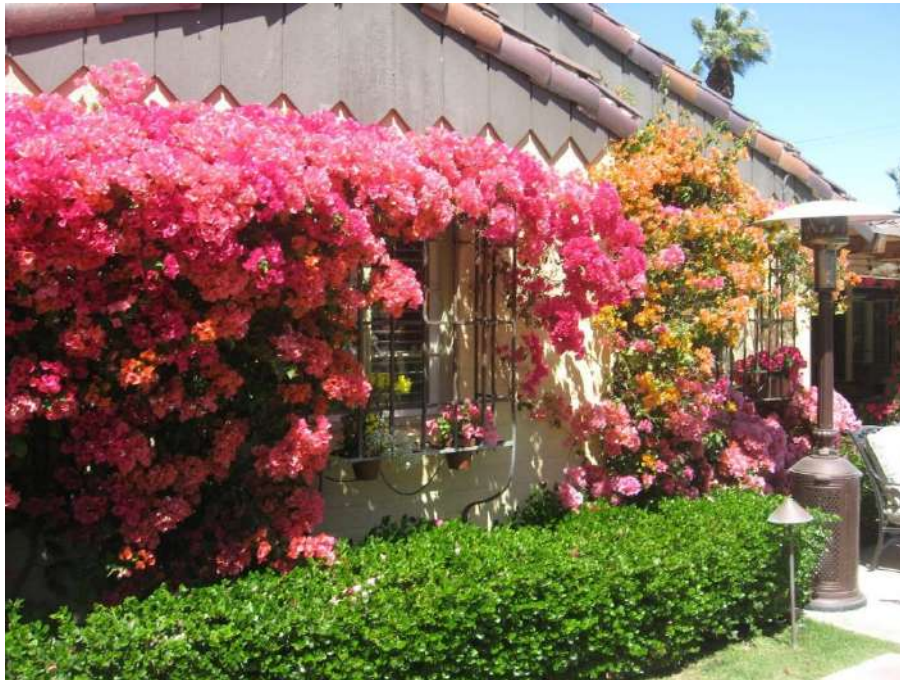
The steel window grilles, designed in traditional Spanish style, are not original features but are period appropriate. (Author photo. July 2023)
